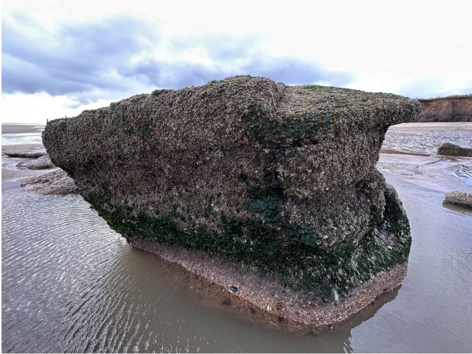
Plate 3-1 Example of the concrete structures found within Landfall 9
